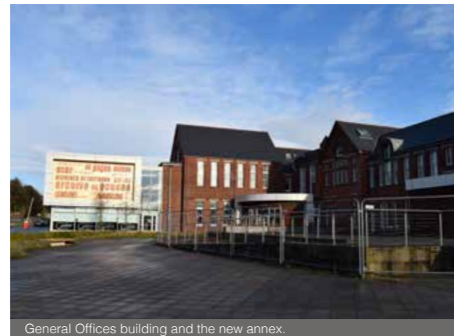
General Offices building and the new annex.
